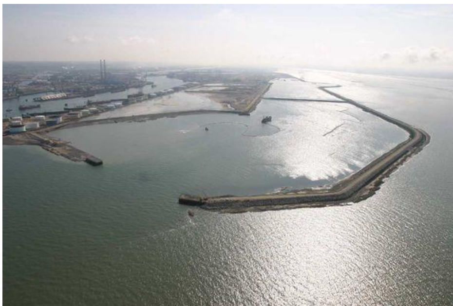
Figure 4.11 The marine wall, protection for both the harbour and the city
