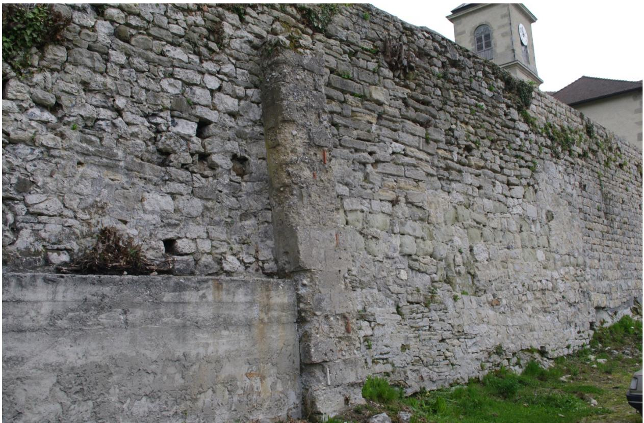
Fig. 4: Multiples phases de construction. Cliché: L. Benoit - SDAHs - CIHAM.
