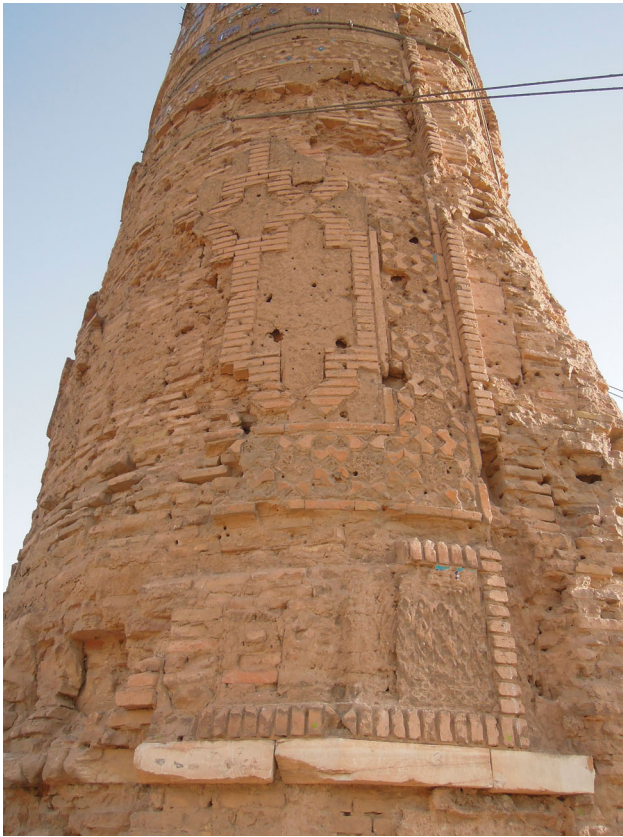
Figure 22. Remains of inset-technique decoration at the bottom of minaret M5 (© S. Aube/Th. Lorain 2015).
