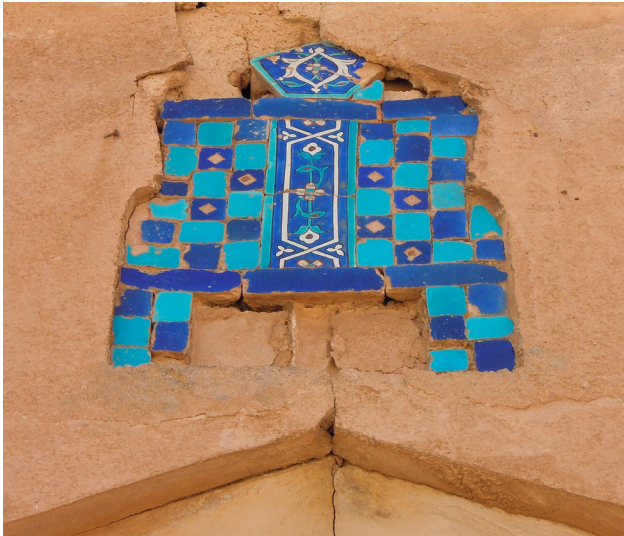
Figure 20. Ceramic tiles replaced above the entrance door of the Mazar-i Zayn al-Din in Taybad (© S. Aube 2015).
