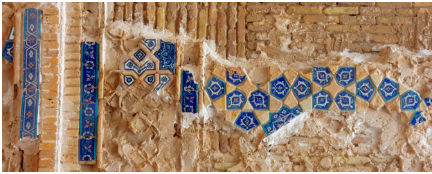
Figure 19. Colored-glaze “cloisonné” tiles and “blue-and-white” tiles from the south-western iwan in the madrasa Ghiyathiyya, Khargird (© S. Aube 2015).
