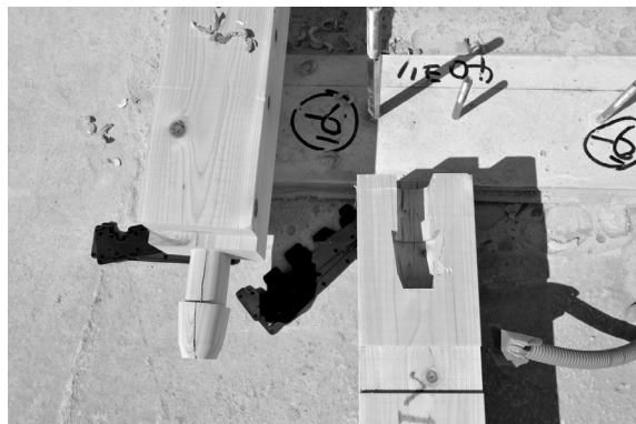
Fig. 18: Mikan, EFEO Centre Kyoto, joints between two beams, September 2013. Photograph ©Benoît Jacquet.
