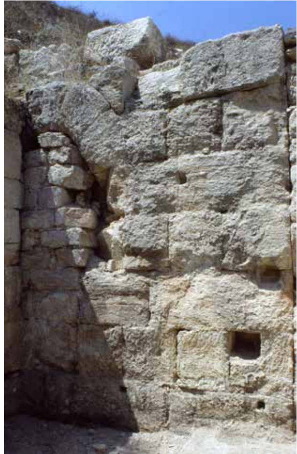
Fig. 9. Abila. Area B. The western wall of the lower room with the blocked arch in 1992 (© A. Michel).
