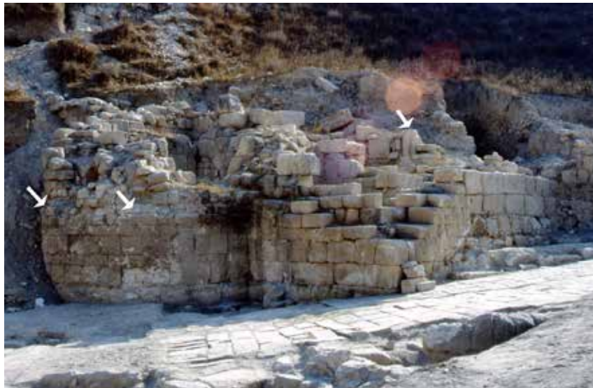
Fig. 6. Abila. The building in Area B. View from the northeast in 1990 (© A. Michel).
