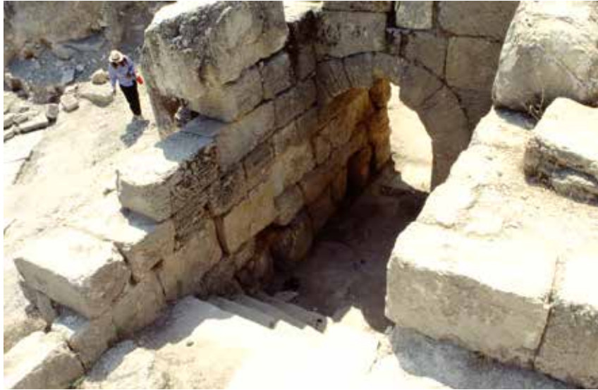
Fig. 5. Abila. Staircase going down to the lower room. View from the north, in the building in Area B in 1992 (© A. Michel).
