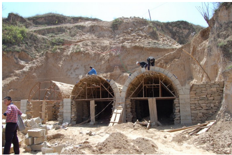
Fig. 11. Building site in Yanchuan district 延川縣, 2011 (©author)
