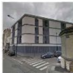
11.19. 112 boulevard Albert 1er © Google street View
