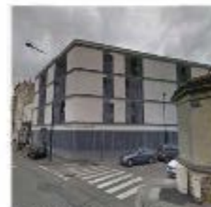
11.19. 112 boulevard Albert 1er © Google street View
