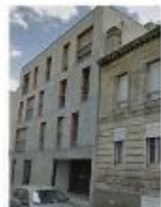
11.17. 118 rue Maube © Google street View
