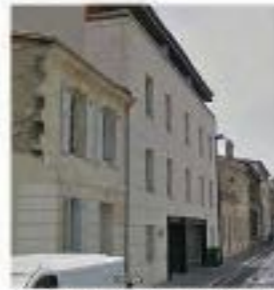
11.12. 30 rue Jean-Daudinville © Google street View
