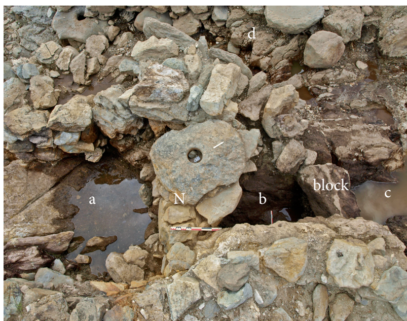
Fig. 15: View of the main features of the mill's hydraulic system: a) undercroft, b) flume and c) head-race. The north wall separates the undercroft from the flume. The flume is separated from the head-race by the block (ST 121-184). The spillway (d) to the west skirts the mill (photograph by N. Minvielle Larousse).
