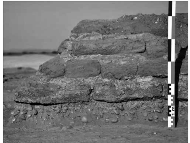
Plate 1. Stratigraphic sequence of pyramid construction (from bottom to top): natural ground surface, layer of sand mixed with pebbles (70 to 120mm), grey mortar (30 to 50mm) and mud bricks.
