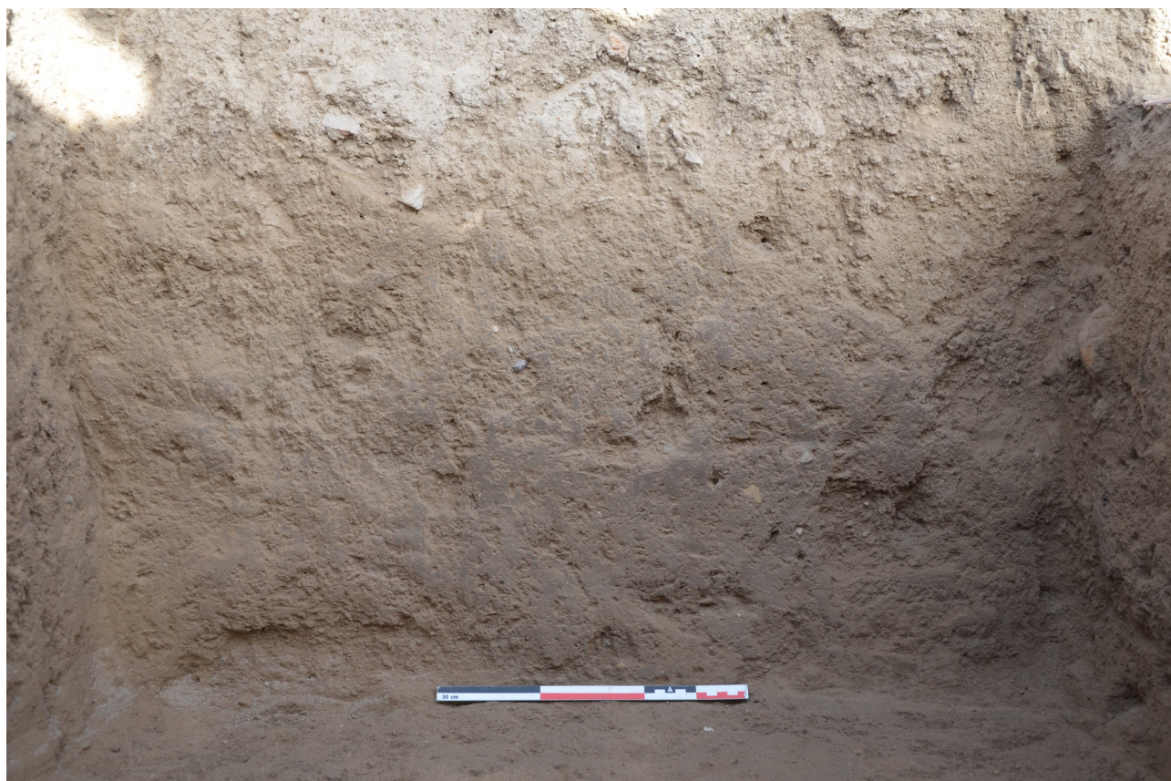
FIG. 6: Compact mud-bricks in the core of the structure 1405 (= 1413) (MAA)
