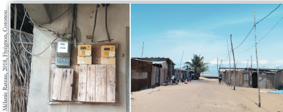
Figure 5. Metres installed in the neighbour's house and DIY connection.
