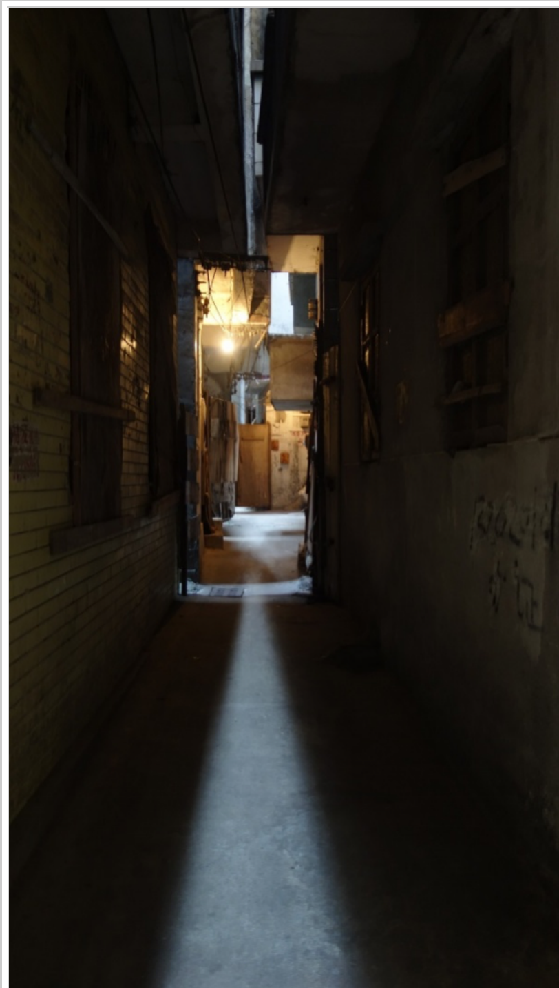
A thread of light between two 'kissing' buildings in an urban village in Guangzhou, Guangdong province. December 2016 Source: AUTHOR. © Cinzia Losavio.
