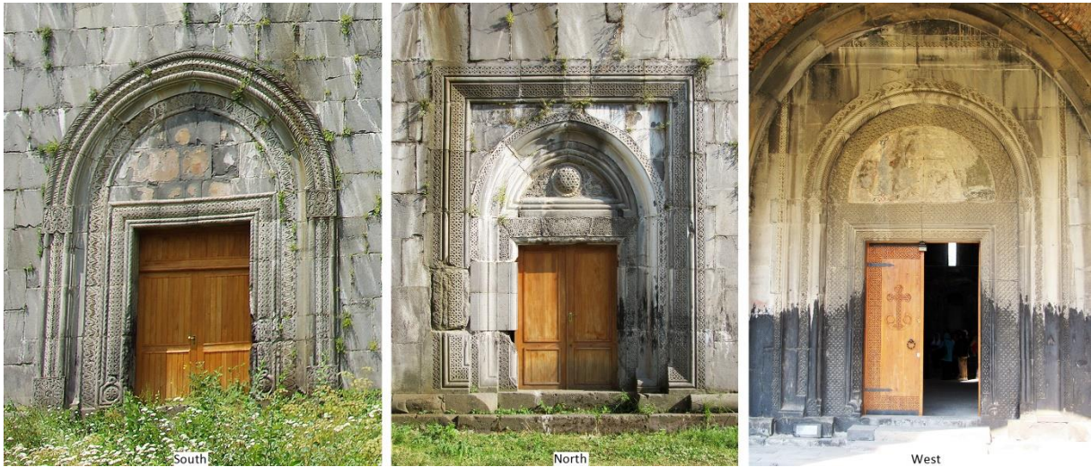
Fig. 18. Pəghəndzahank/Akhtala. South, north and west portals of the main church (Photos: Patrick Donabédian)
