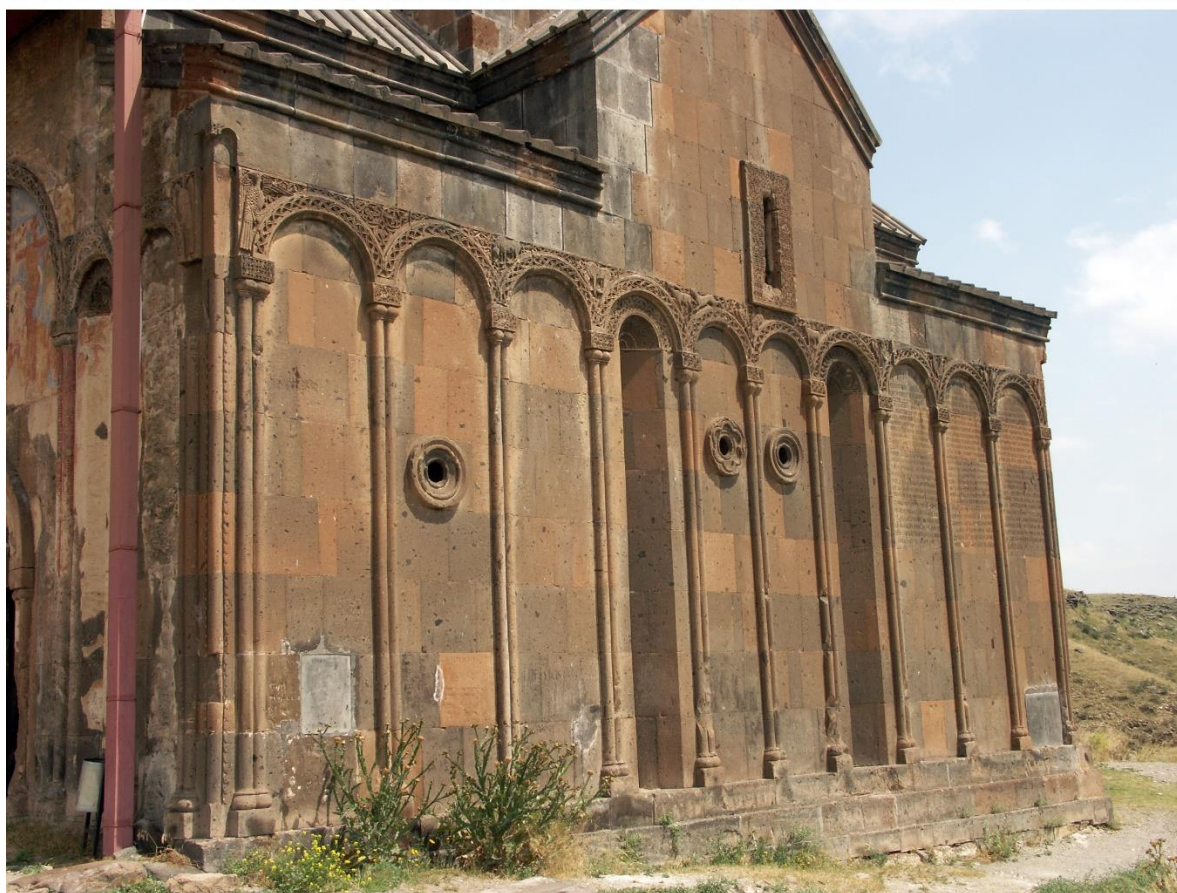
Fig. 5. Ani. St. Gregory of Tigran Honents. Blind arcade-colonnade on the south façade (Photos: Patrick Donabédian)
