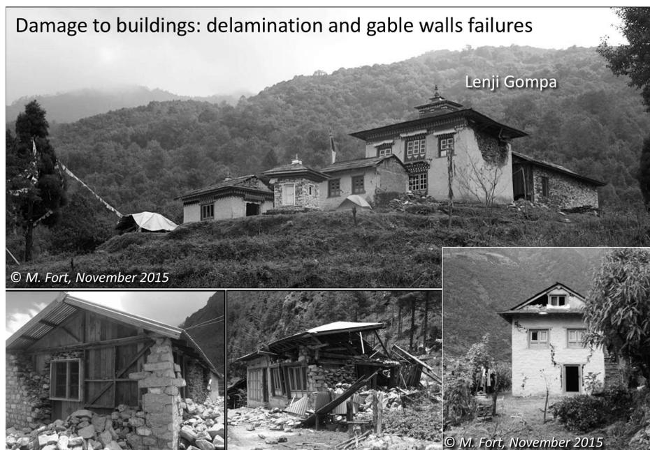
**Fig. 11: Significant damage to buildings (Lenji Gompa and houses) in the Khari Khola catchment. “X-cracking” and gable wall failures both due to the type of building and to colluvium soil being susceptible to shaking. (Photos: © M. Fort, November 2015)**
