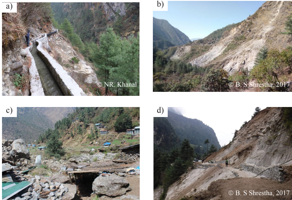
Figure 4: Earthquake induced hazards losses and damages in study area. a) Canal damage at Manjo by landslide b) landslide induced at Nackchung village c) Destroyed stone masonry building and collapse crops and cultivated land at Surke village south of Lukla, d) Trail damage by Landslide north of Phakding.
