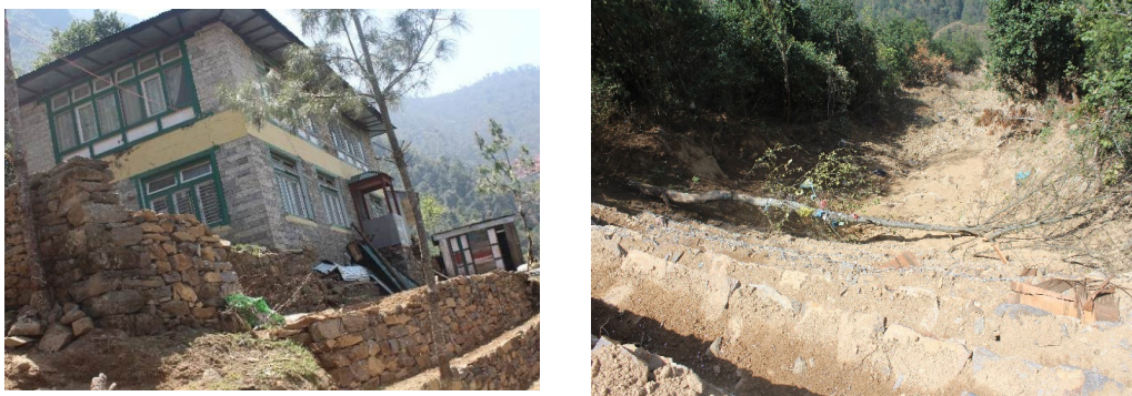
Figure 5: Wall constructions to mitigate house and trail at Surke village a) landslide affected house upper part b) wall construction (stone and mud) to control headward extension of landslide.
