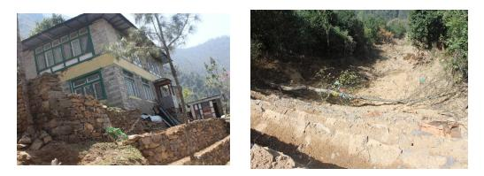
**Figure 5**: Wall constructions to mitigate house and trail at Surke village a) landslide affected house upper part b) wall construction (stone and mud) to control headward extension of landslide.
