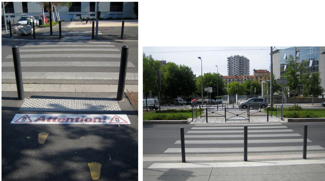
Fig. 2 & 3 - Two examples of ‘bateaux’ and hazard warning strips at pedestrian crossings
