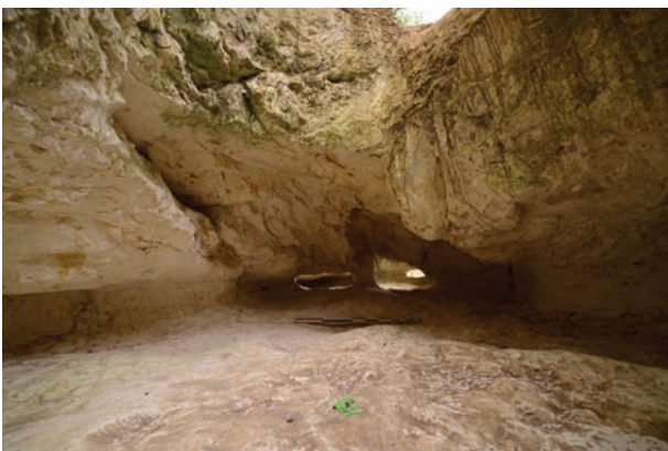
Fig. 5 – Vert-la-Gravelle 'La Crayère'. Interior of the bell-shaped shafts 1 and 2. View of Pit 2 in the direction of Pit 1. A pillar was left between the pits, in order to buttress the mining area. Some retained pillars are also observable. Photo R. Martineau.
