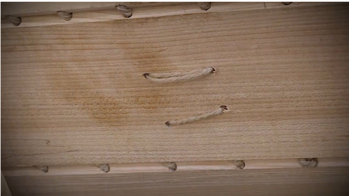
II.69 Pogled na vanjsku oplatu i rupe za vezanje View of the exterior side of the planking and the holes for lashing the frame (fotografija / photo by: M. Račan)
