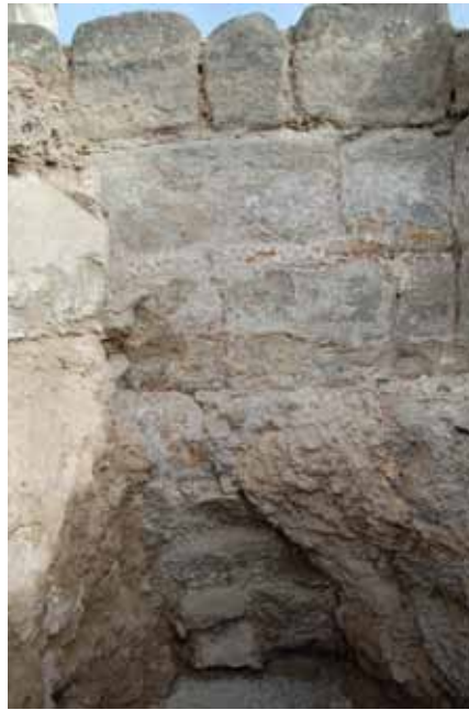
Fig.21: Detail of the foundation under wall M4 in B2 after having removed the mortar (JB 2014).
