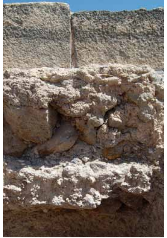
Fig.47: Detail of the different layers of the foundation in sounding G2 (JB 2014).
