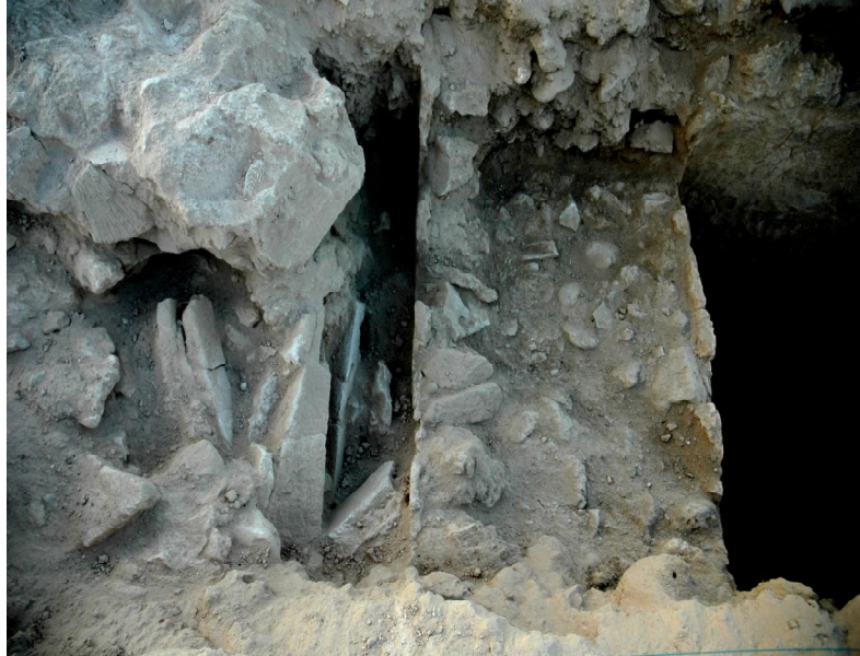
The third compartment (S9), with the collapse from the superstructures of the mosque inside the basement
