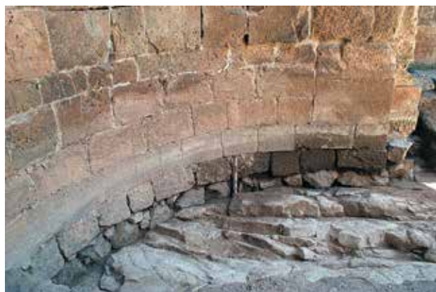
Fig. 4. Yereruyk basilica. Foundations of the south part of the apse (Photo: D. Martinez, LA3M, 2013).
