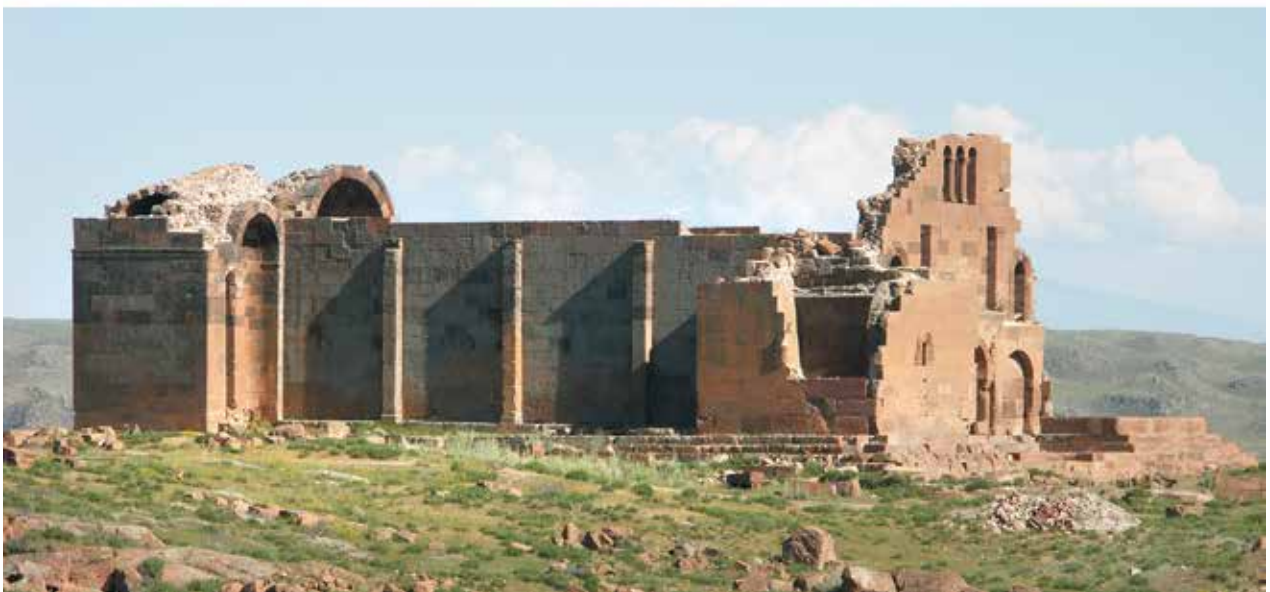
Fig. 2. Yereruyk basilica. General views from south-west and north-west (Photos: Author, LA3M, 2011 – 2014).
