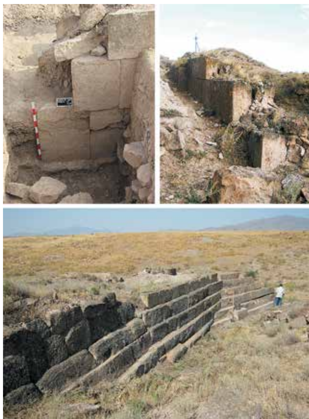
Fig. 18. Yereruyk. “Dam”. North face of the two north walls: the middle wall, at the top and the one upstream, at the bottom (Photos: Author, LA3M, 2015).
