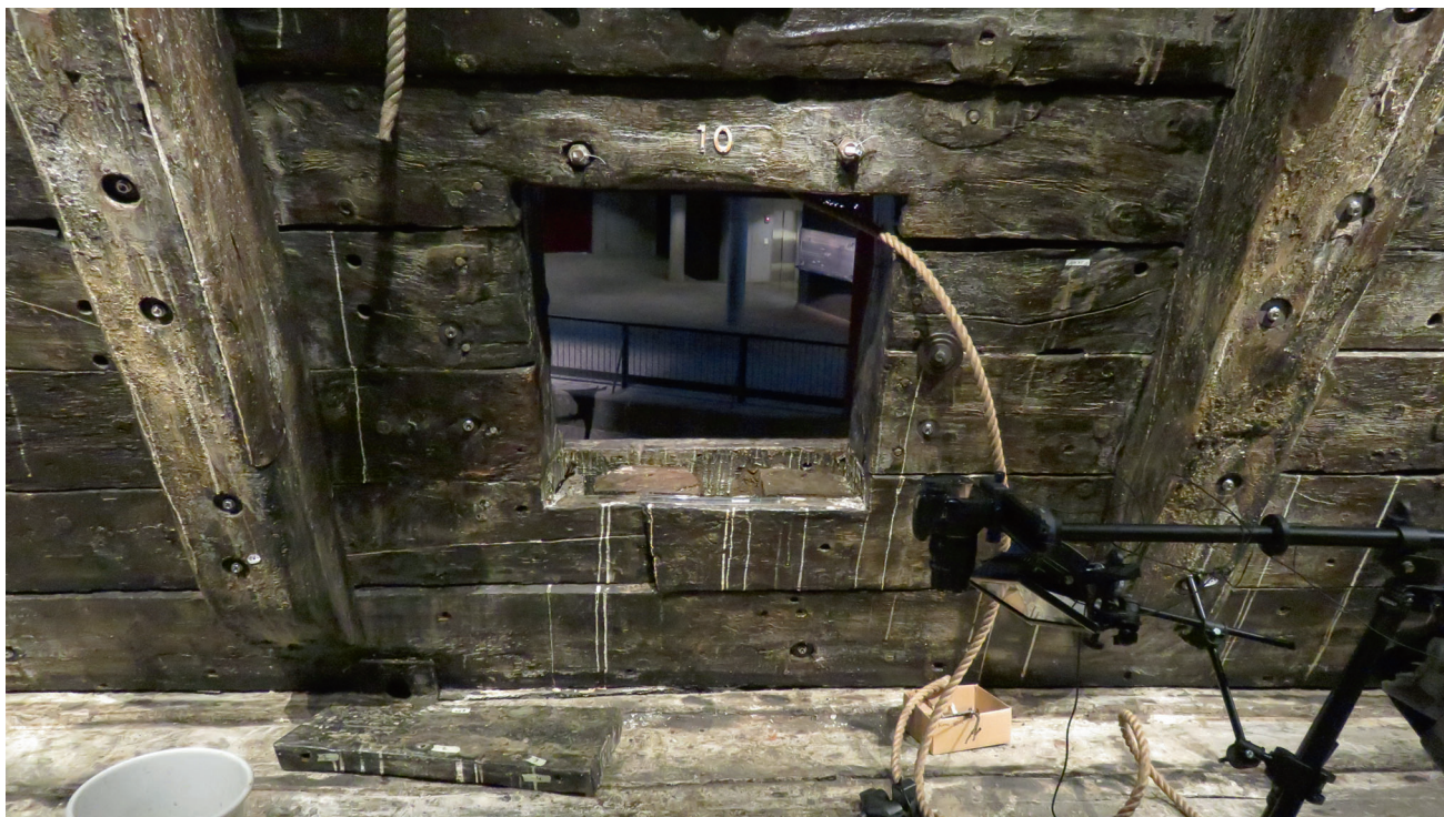
Fig. 1: One of the gunports on Vasa : access to the end grain of hull planks and ceiling planks is possible. Furthermore, when the oak sill is removed (it can be seen lying on the deck) the cross sections of the sill and the frames can also be accessed (photography A. Daly).
