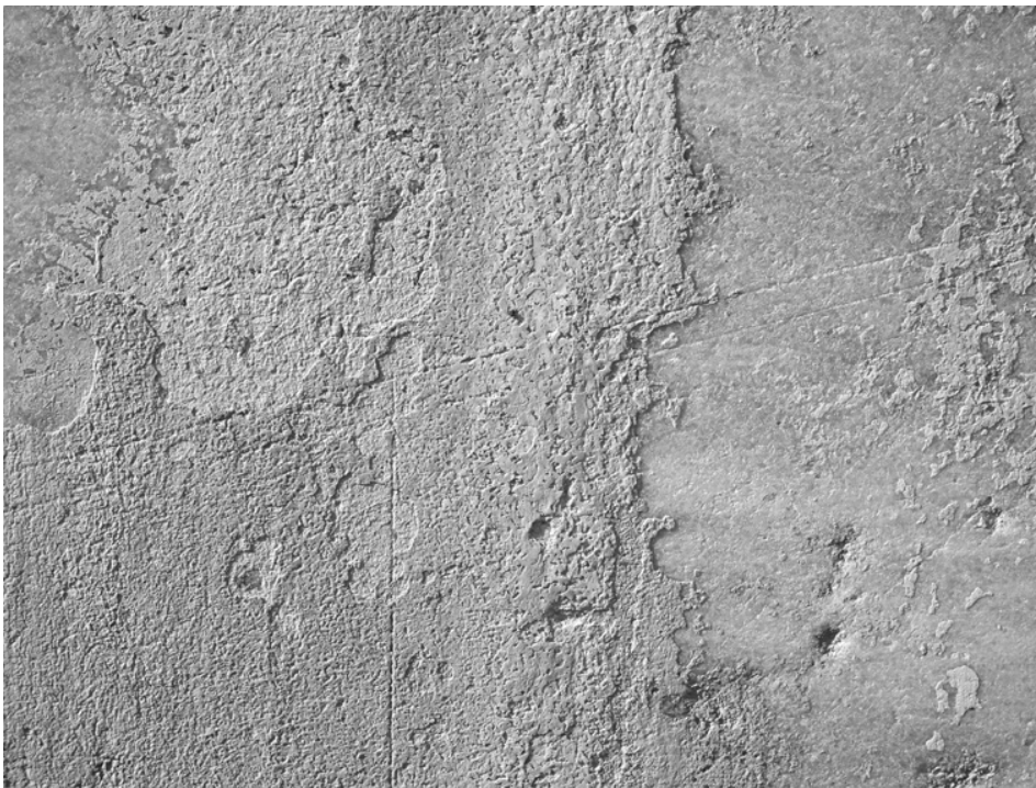
FIGURE 3.1 Ephesos, Upper agora, basilike stoa , vertical and oblique lines incised in a coat of paint. The “blueprint” is visible on the surface of the marble
