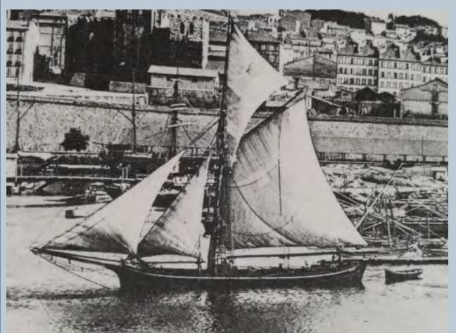
used to cargo goods have a more important rigging, composed by a main mast ("mestre"), a little beyond the master frame, and a other one called "trinquet", at de bow of the ship, with a 25° inclination.
