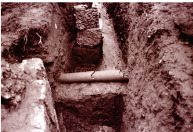
Figure 21: Terracotta pipe passing through the wall C at Fețele Albe (from Daicoviciu et al. 1973a, Fig. 3).
