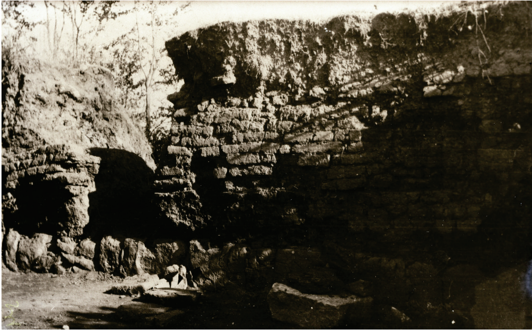
Figure 7: Mud brick elevation at tower no. 1 from Costești-Cetățuie fortress (from Teodorescu 1930, Fig. 8).
