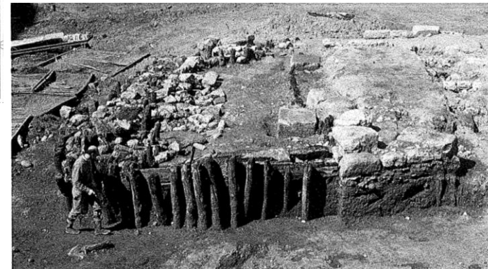
Quay F28. Jules-Verne excavations (M. Derain / AFAN)
