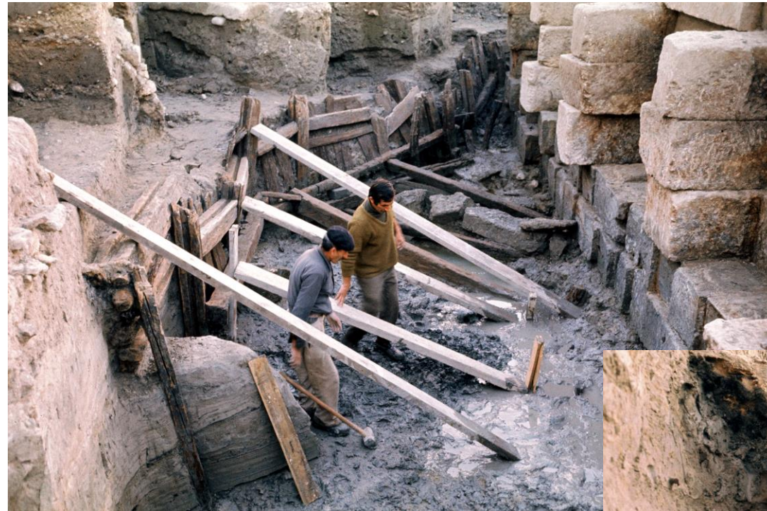
Cofferdam system of the freshwater bassin (© Antoine Chenet, CNRS-CCJ, 1972)
