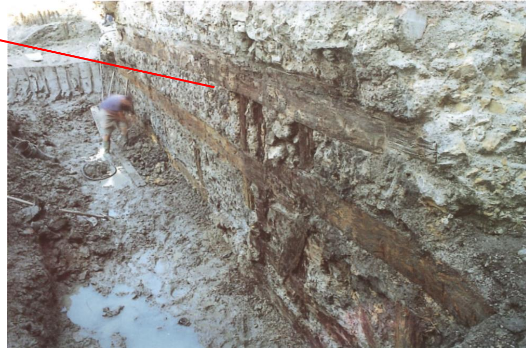
Roman wharf made with limestone and Pozzolan foundation. Jules-Verne excavations (M. Derain, 1999)
