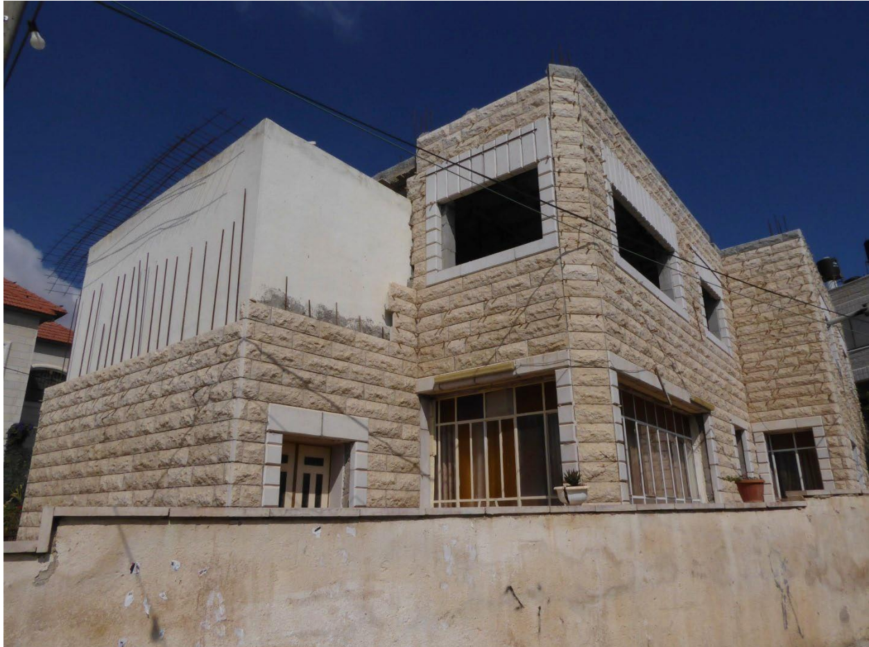
Image 57 Kafr Malek: Concrete and iron reinforced masonry (photo RC).
