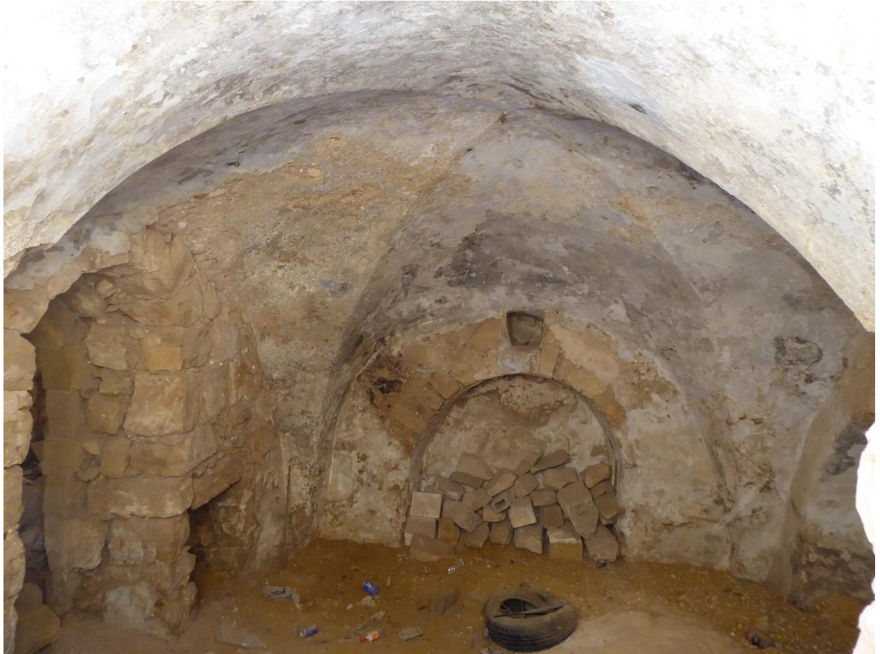
Image 61 Hebron's old town: cross vault in an abandoned building. We can see the importance of corners in load bearing issue.
