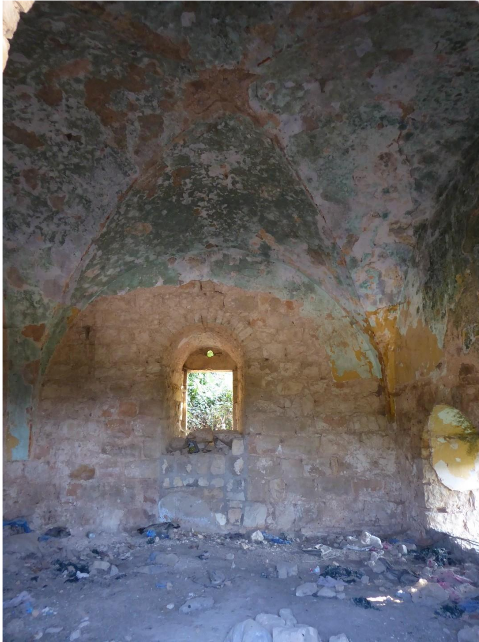
Image 16 Birzeit compound: Cross vaults ending with pointed vault interior traditional hall
