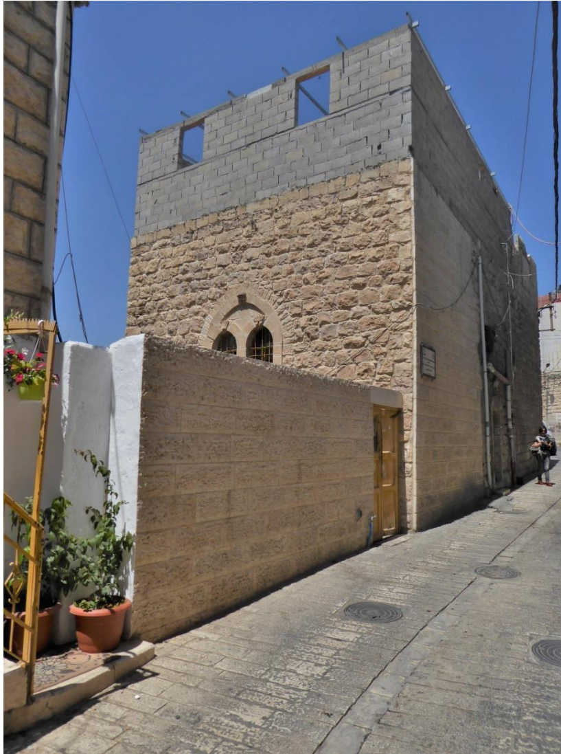
Image 56 Hebron: A restored building. Several kinds of stones in this building; undressed stones seen in the wall with arched window and new dressed stones (hadjar imsams) facing the street. At the upper level, we can see some concrete blocks .... (photo RC)
