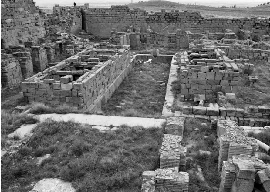
Fig. 11. Timgad, basin of the Byzantine fortress viewed toward the north. Note the overflow indicated by an arrow. (Xiaotong Gao, 2015, CC BY-SA 3.0.)
