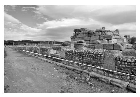
Fig. 9. Sbeitla: raising of the threshold testifying to the elevation of the street level. The upper parts of the wall are restored. (N. Lamare, 2019.)
