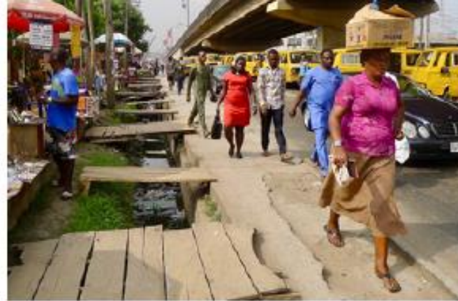
Risky open drains
