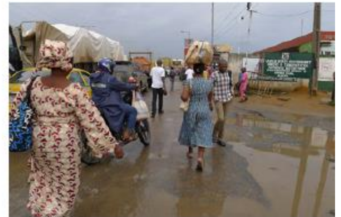
Lack of storm water drainage
