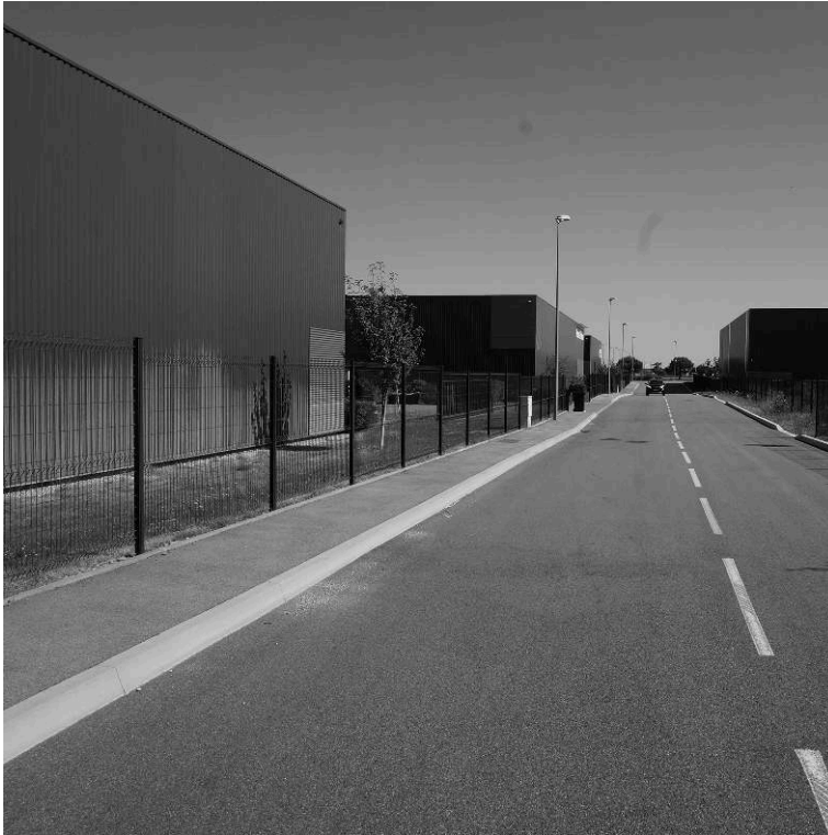
Figure 3; Uniformity and horizontality of current urban forms in business parks (C. Charieau, 2018)
