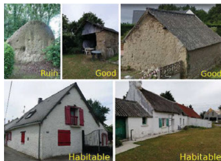
Fig. 7. Cob buildings in different states of preservation
