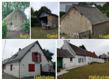
Fig. 7. Cob buildings in different states of preservation
