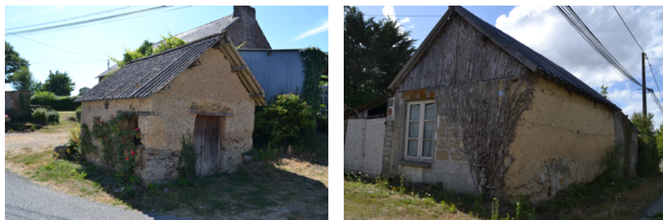
Fig. 02. Examples of raw earth constructions in the Fégréac and Chevallerais cities ©M. Miranda
