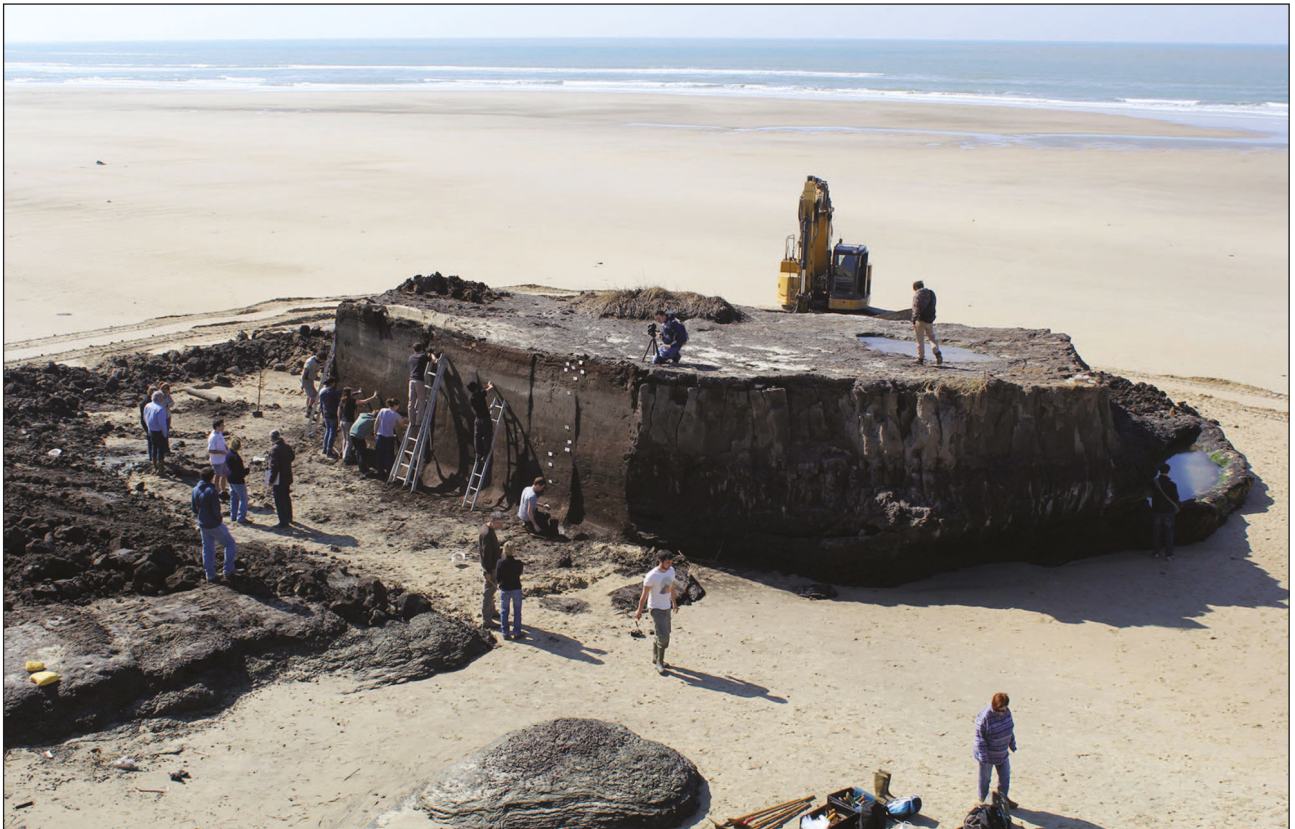
Fig. 5: La Lède du Gulp, first survey and sampling campaign in March 2014 (photo N. Prévôt).
