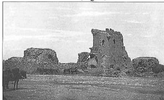
Fig.7. Tower of Constantine before the restoration [38]
