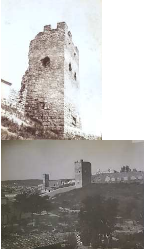
Fig. 10. The Crisco tower before the restoration and after [32]
