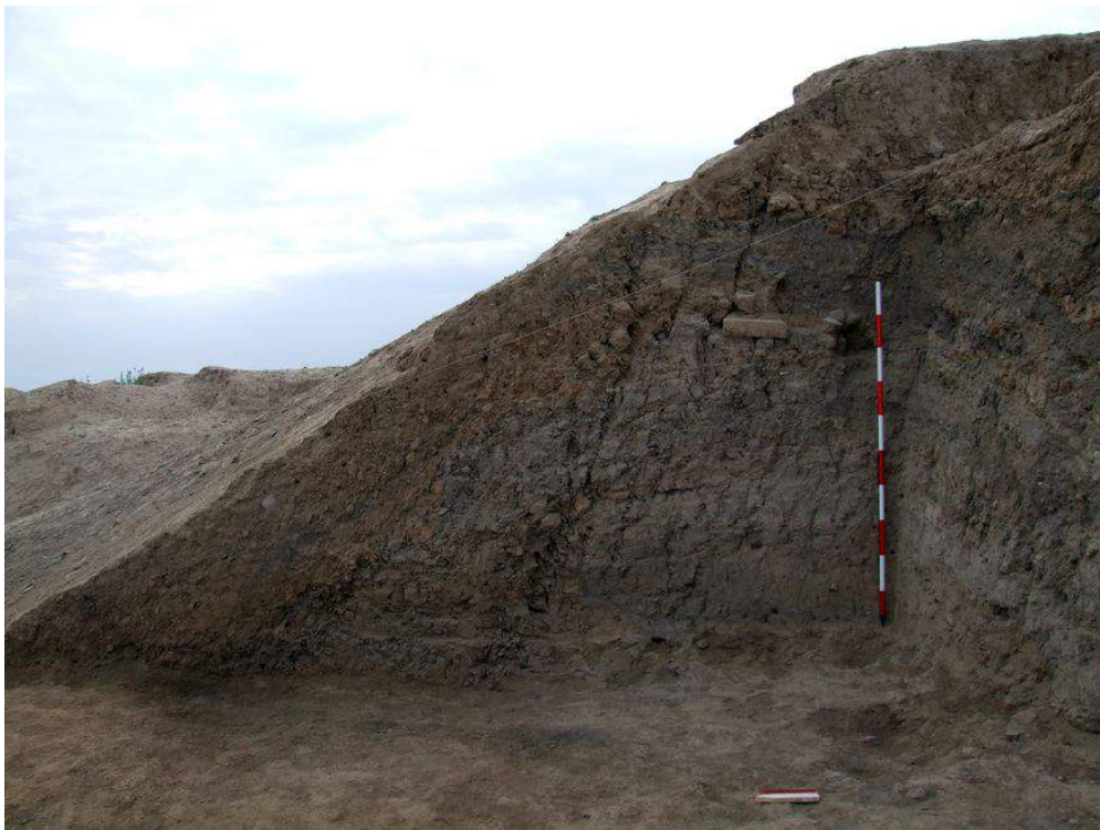
Figure 14: Southern part of the Eastern section in Area B showing the listric faults, 2013 (© MAFQS, photo by J.-J. Herr).
