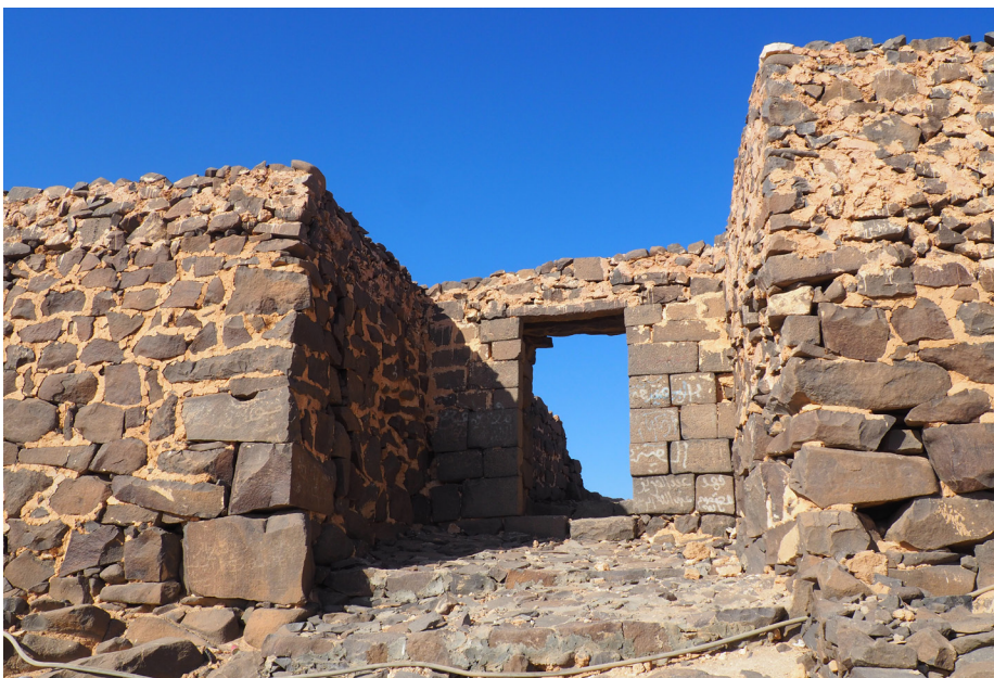
Fig. 11. The gate, from outside of the citadel (P.-P. F. 2021)
