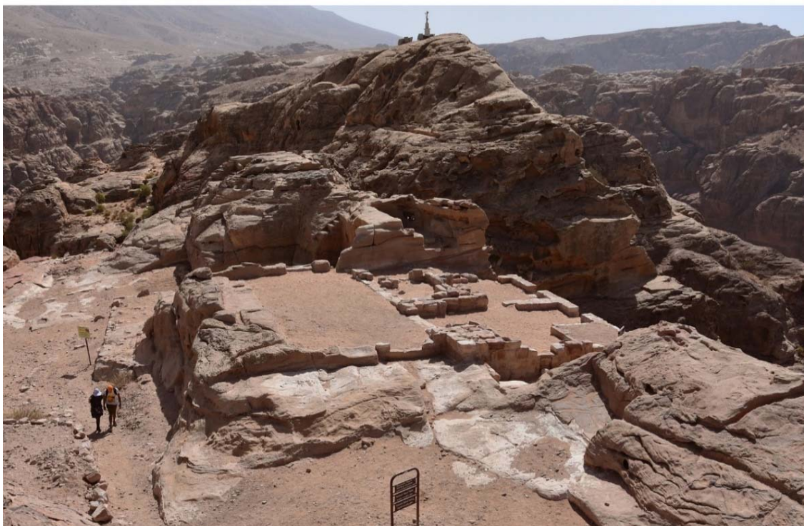
Figure 4. The bath building from the north, before excavation (top) and after excavation and preservation works, in 2016 (N. Paridaens).
