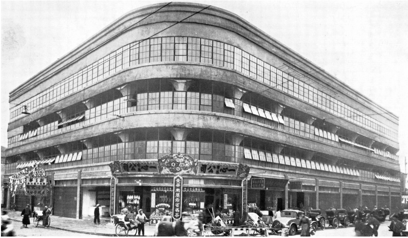
Figure 4.8. Foochow Road Market, Shanghai, 1930. Report for the Year 1930 and Budget for the Year 1931 , Shanghai Municipal Council. Courtesy of the Virtual Shanghai Project. Located in the Central District of the International Settlement, Foochow Road Market was built to relocate the dealers from the old Maloo Market. The building was equipped with a lift, cold storage in the basement, and water-flushed latrines for both sexes.
