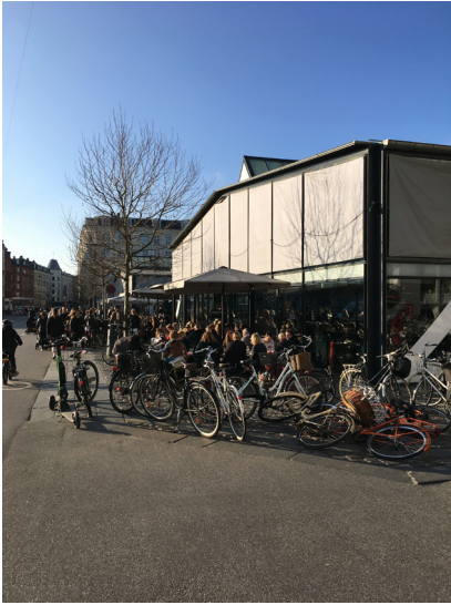
Figure 10.7. Torvehallerne, Copenhagen. Photograph by author, March 29, 2019.
