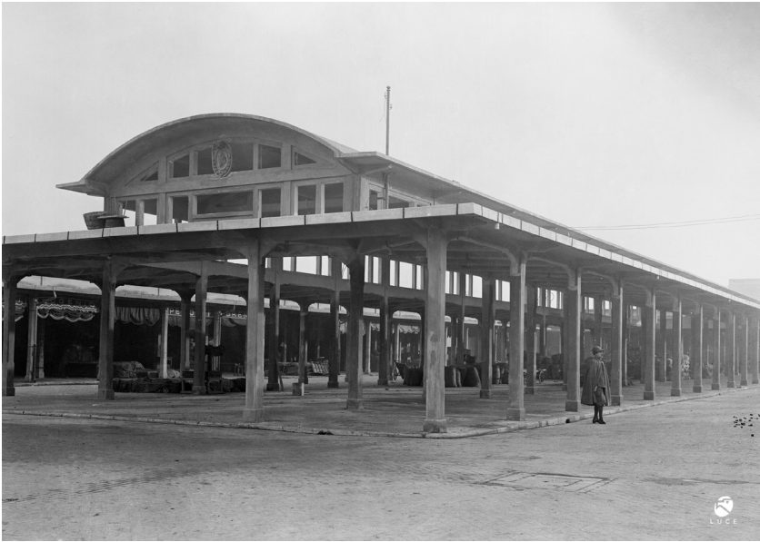
Figure 8.6. Reinforced concrete stalls at the Wholesale Market, Rome, 1926. Emilio Saffi, architect. Courtesy of Archivio Luce.
