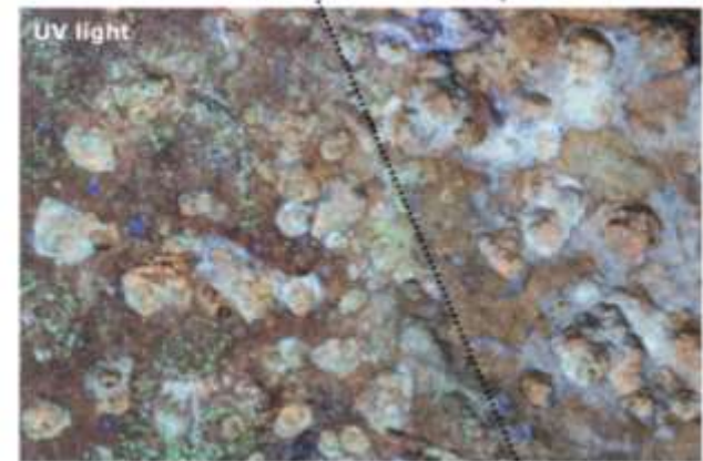
Photographs of the flaking zone under white and UV light (Quiers et al., under review)
