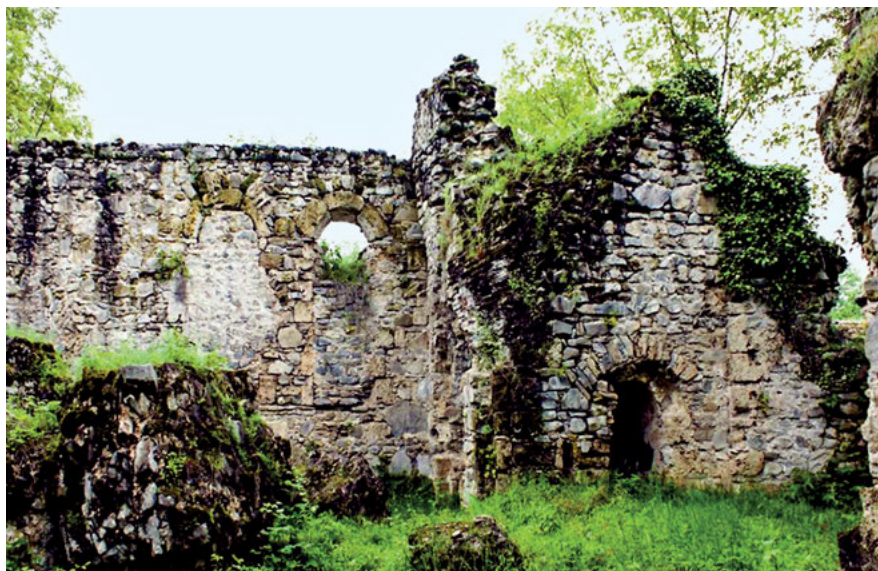
Fig. 8: Yeddi Kilsə. Western church. North wall and northeast sacristy seen from the south.
