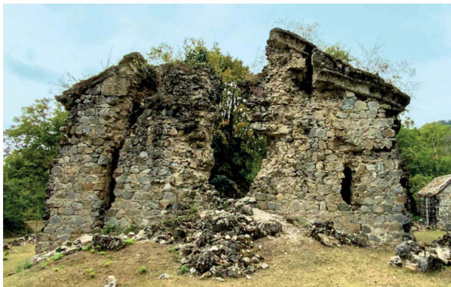
Fig. 19: Yeddi Kilsə. Eastern church. East façade.
