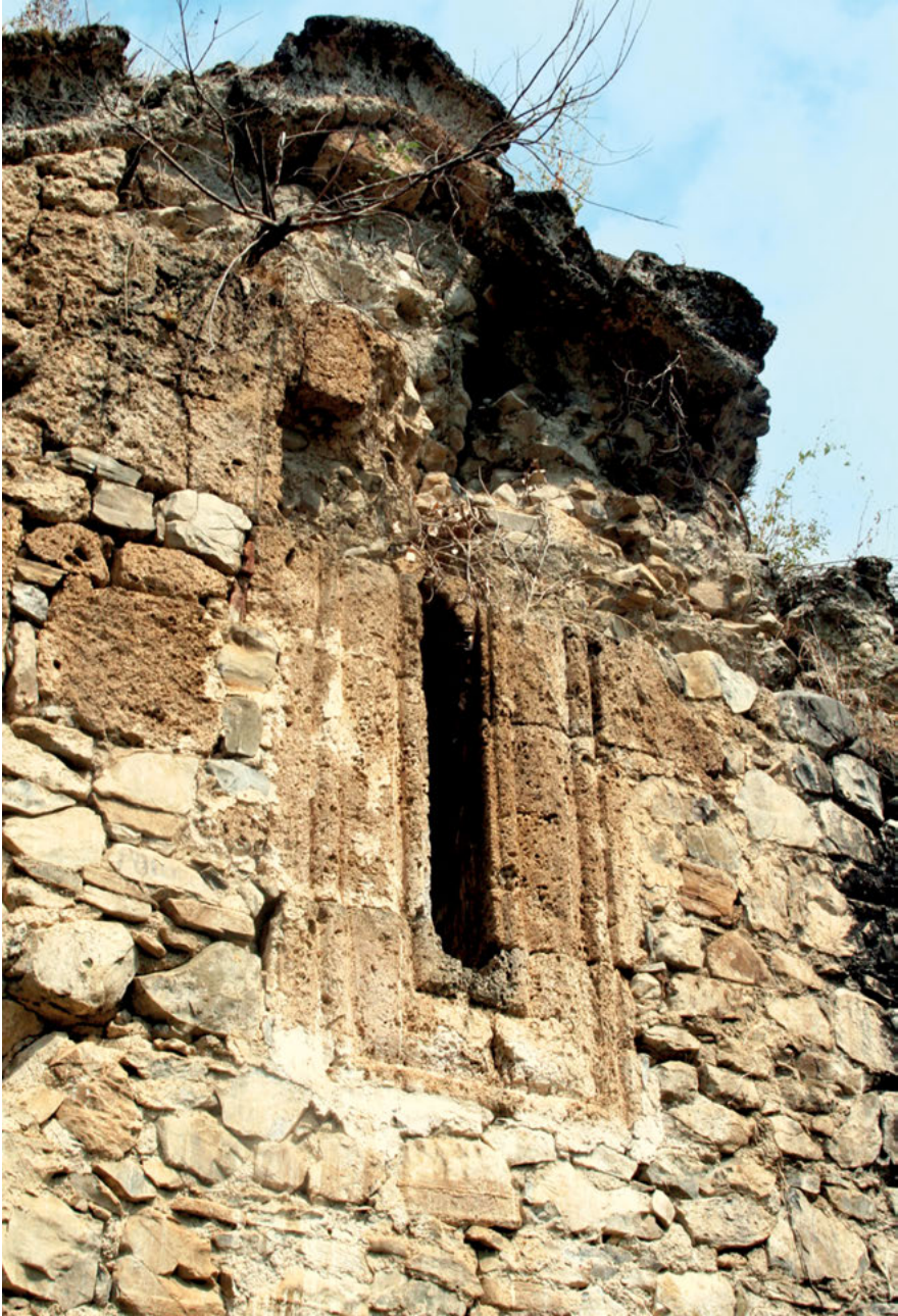
Fig. 21: Yeddi Kilsə. Eastern church. Central window of the south façade.
