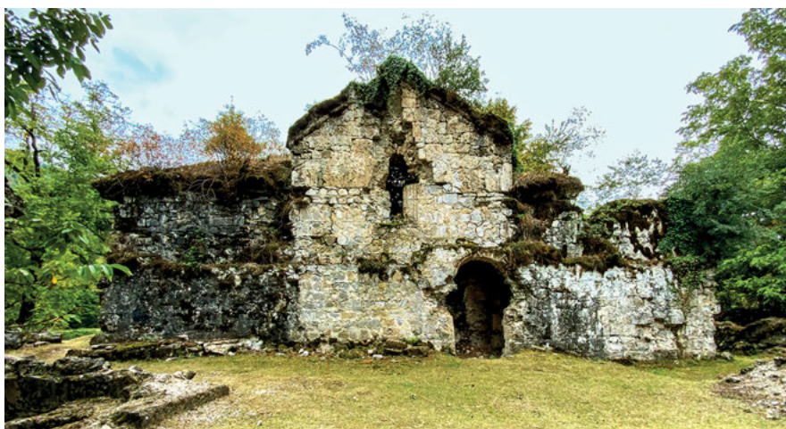
Fig. 18: Yeddi Kilsə. Eastern church. North façade.
