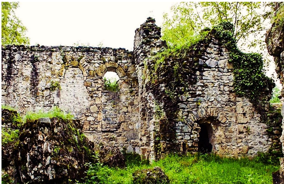
Fig. 8 (p. 399). Yeddi Kilsə. Western church. North wall and northeast sacristy from the south. Online photo Sefer Azeri.
