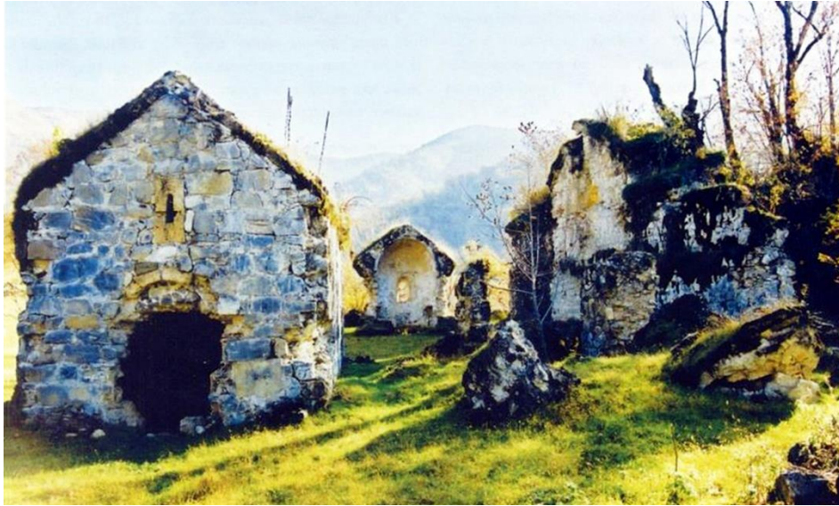
Fig. 24 (p. 419). Yeddi Kilsə. Three chapels to the north of the eastern church. Photo Mamedova (2004: 152, fig. 85)
