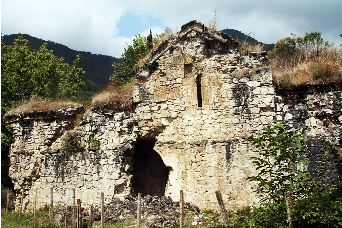
Fig. 17 (p. 410). Yeddi Kilsə. Eastern church. South façade.
