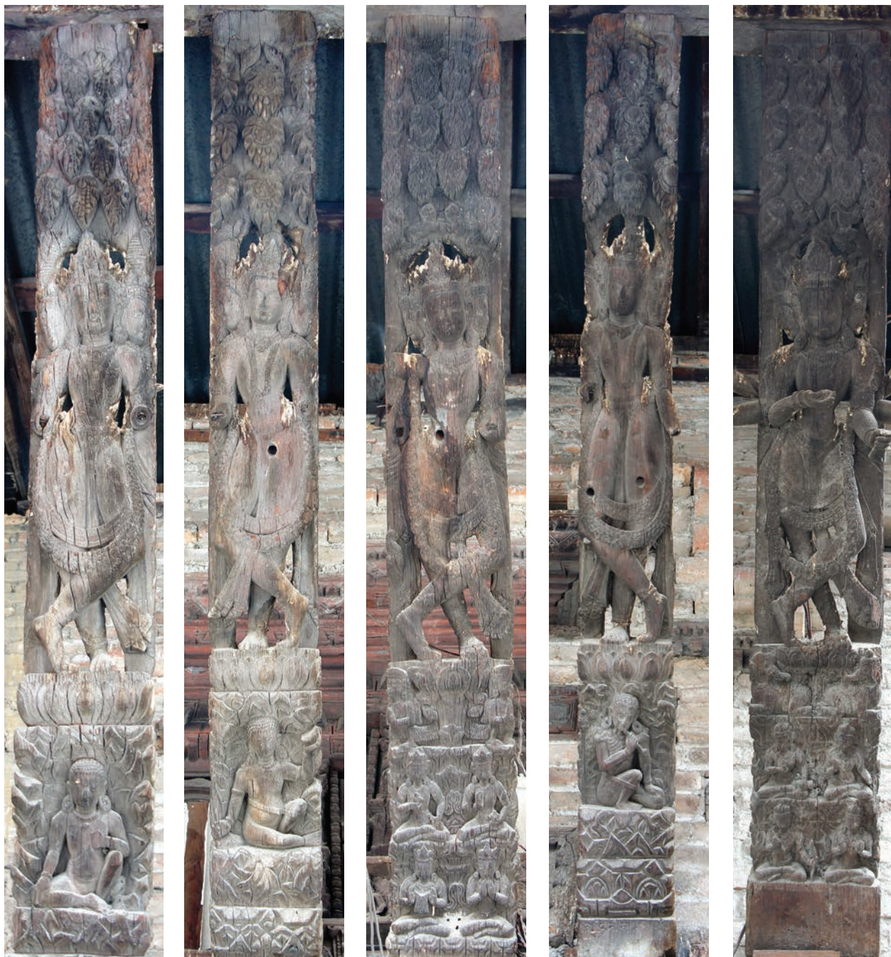
Existing struts of Itumbáhah East Wing courtyard facade. Photographs October 2013
