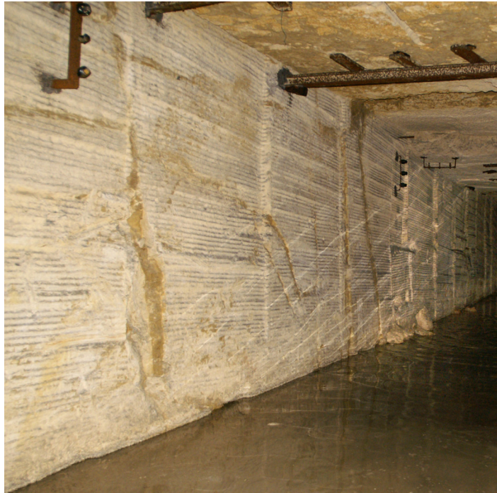
Figure 8: Quarry wall with tool marks from roadheaders with rotating drill bits – Roches & Carrières Archives.
