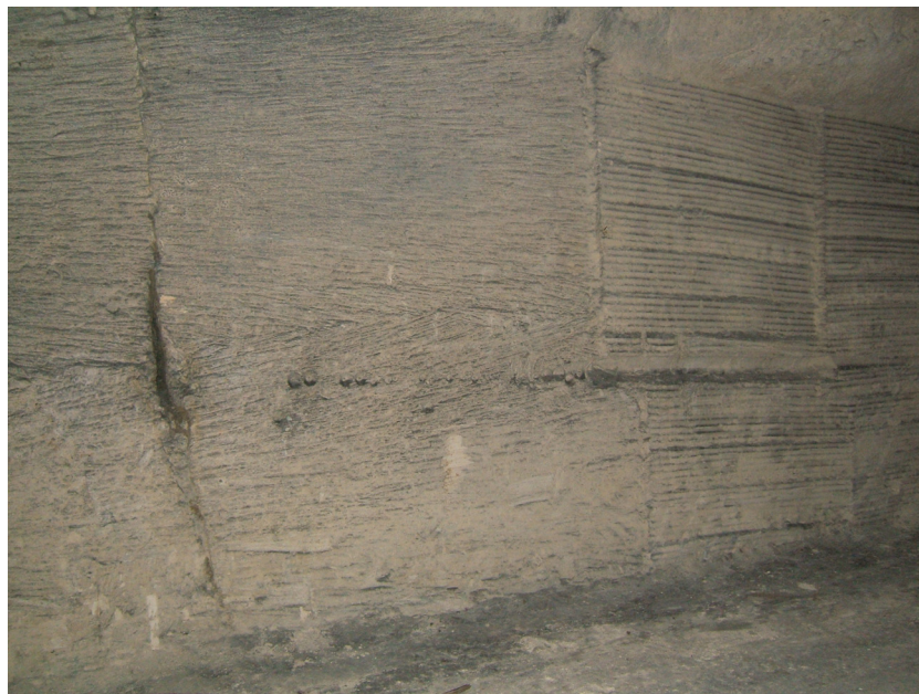
Figure 3: Tool marks of lance (on the left) and rotating drill bits (on the right) – by J-P. Gély.
