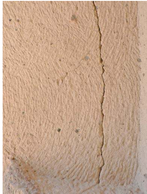
Fig. 14 West wall of the nave of the church Göreme n°4b, radial and slanted cutting by short-handled pick (A. Lamesa).
