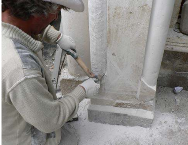
Fig. 18 K. Manap using the polka as a scraper (A. Lamesa).
