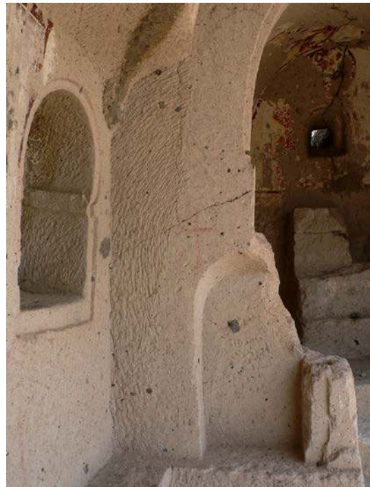
Fig. 13 View of the east wall of the nave: junction between the short-handled picks' tool marks and the polkas' tool marks (A. Lamesa).
