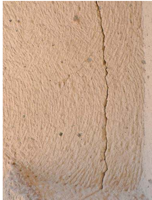
Fig. 14 West wall of the nave of the church Göreme n°4b, radial and slanted cutting by short-handled pick (A. Lamesa).
