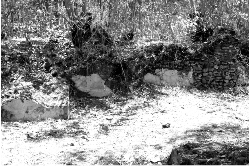
Susinyos bath (foundations of the pavilion)
