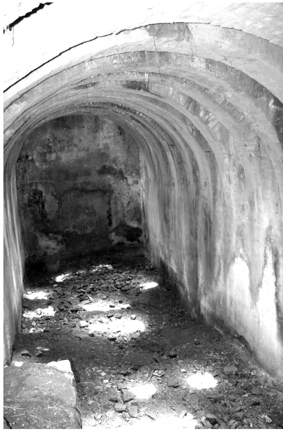
Susinyos Palace (arched cistern)
