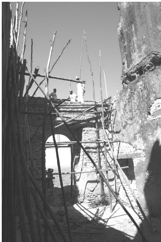
Guzara castle (interior view during the consolidation work)
