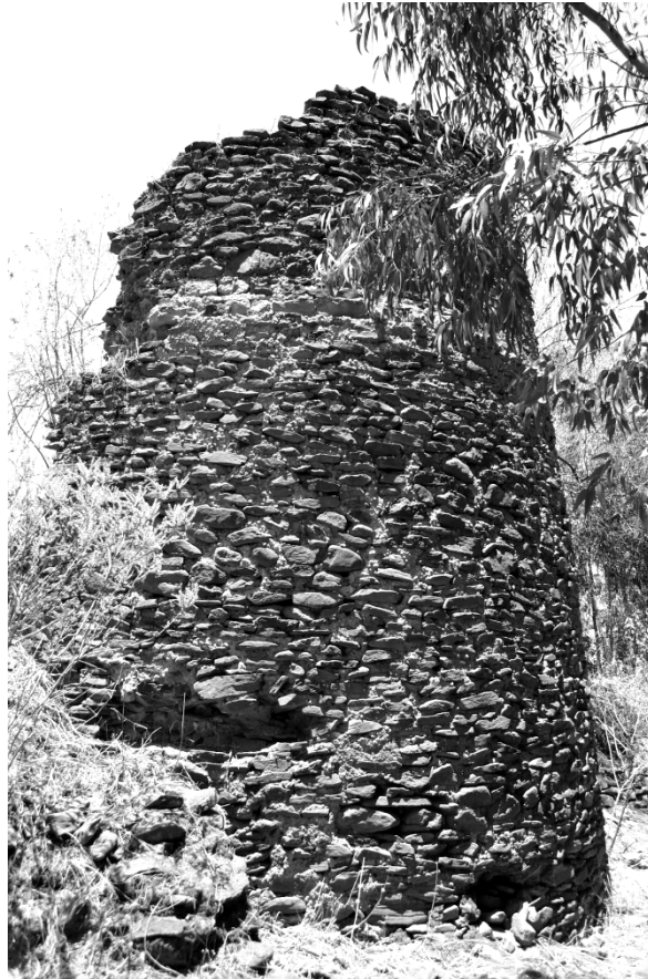
Susinyos castle (southeastern tower)
