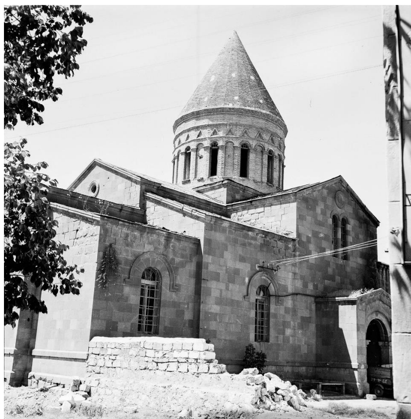
Fig. 3.4. Church of Surb Gēworg (1869), city of Nakhichevan, view from the northwest. Photo: A. Ayvazyan (1960), УИОТС v-21391, Argam Ayvazyan's Fund
